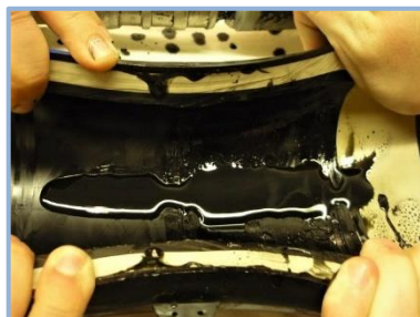
Contaminating fluid inside joint/cable interface
