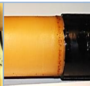
Jagged/ non-radial semicon cutback with evidence of insulation surface erosion
